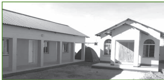
The first phase of the Omakuva building project is completed: the sister's house includes a small chapel, office rooms, kitchen and dining room.
